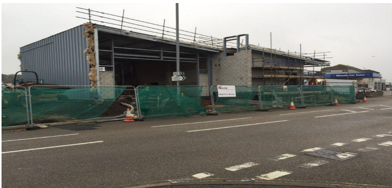
Hayle, Tri-partite Emergency Services Base in construction, 2015
