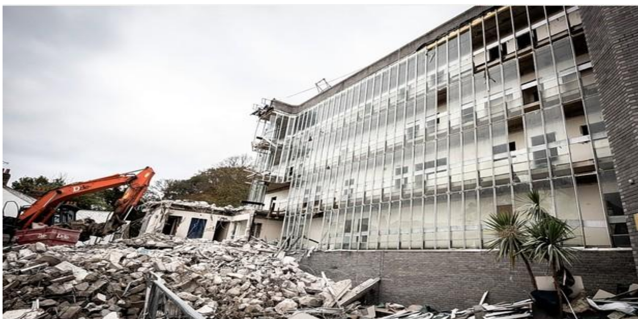
Truro Police Station, demolition of Tregolls Road 2015
